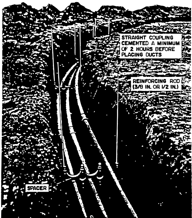
Fig. 3 - Partially Completed Bend
